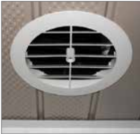
EZSoffitVent installed
