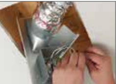
Connect the wiring and attach duct to installation adapter
