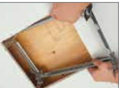
Insert single-hinged Flex-Z Fast® installation bracket
