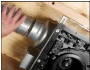
Attach 4" or 6" duct to the fan's duct adaptor
