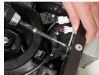
Unscrew & remove junction box and duct adaptor from fan
