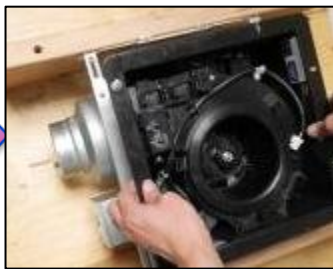
Insert housing containing the motor assembly into the center of the bracket
