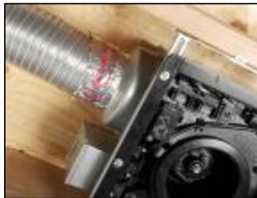
Secure the connection using qualified tape
