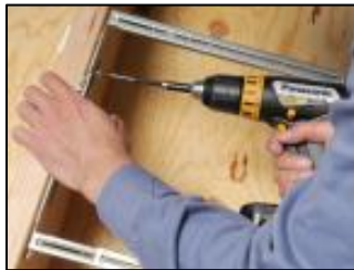
Secure bracket to joist by screwing in all 4 sides of bracket
