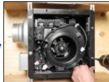
Screw the housing's metal flange to each connection point on the bracket
