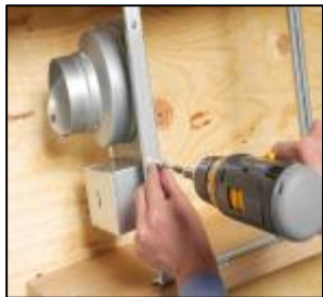
Screw the junction box and duct adaptor onto the bracket
