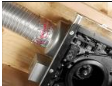
Secure the connection using qualified tape
