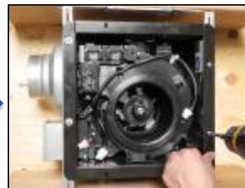
Screw the housing's metal flange to each connection point on the bracket
