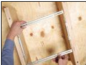
Position the Flex-Z Fast™ bracket in between the joist
